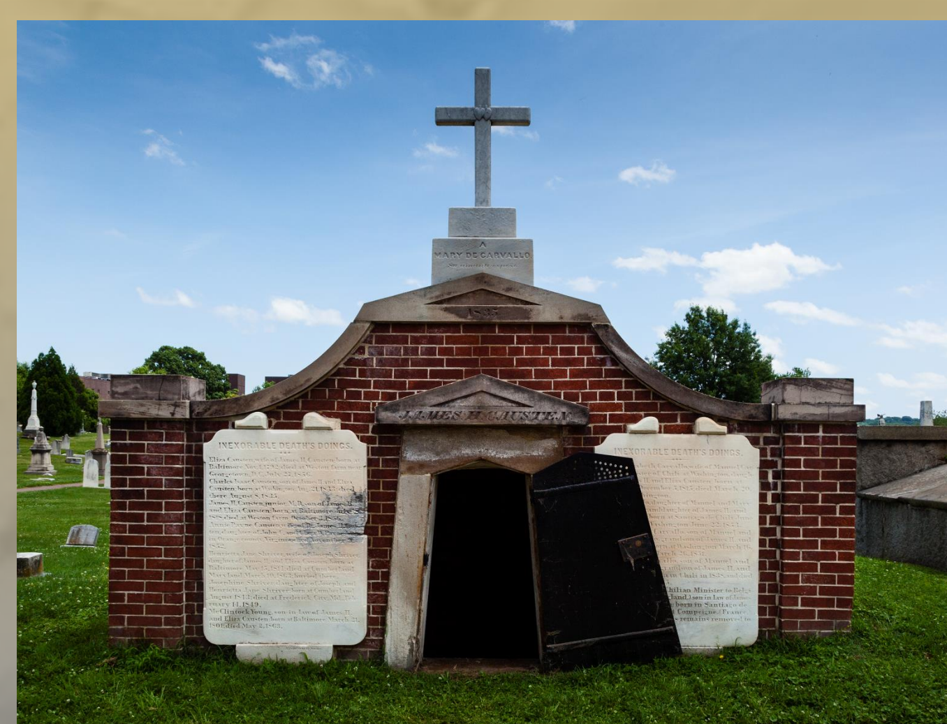
Figure 1. Exterior of the Causten family vault.
